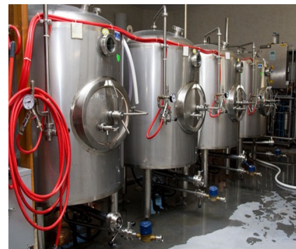
Beverage processing plant production line
